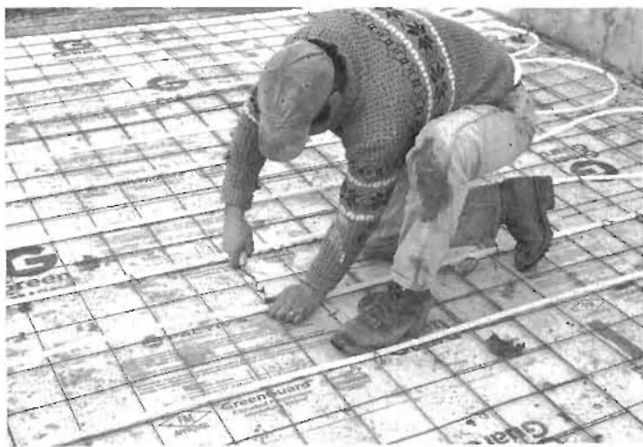
Fig. 4.6: Steve Bedard fastens his polyethylene tubing to the wire mesh with a special rotating hook made for twisting tie bands.
