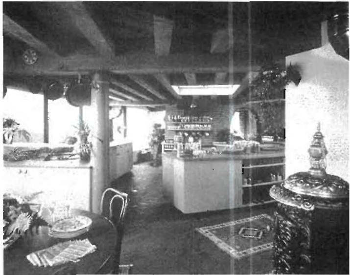
Fig. 1.6: Heavy timbers support a 15" to 18" thick earth roof at Baldtop Dugout in New Hampshire, designed by Don Metz.
