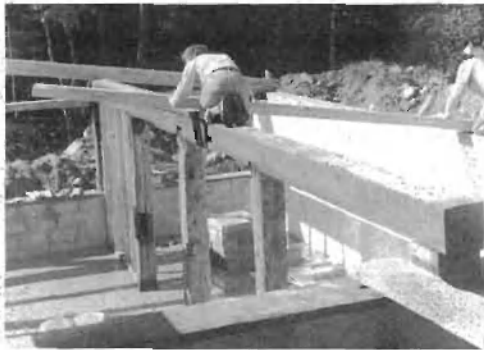
Fig. 6.8: We slide a rafter along the girders.
