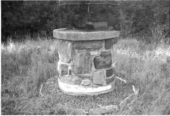
Fig. 11.3: Any projection through the earth roof – skylight, chimney, vent stack – should be surrounded by good drainage material, such as #2 crushed stone.
