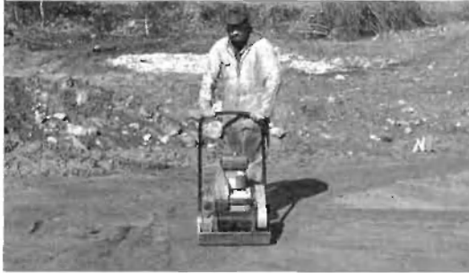
Fig. 3.4: Dennis Lee tamps the sand pad at Earthwood with a power compactor.
