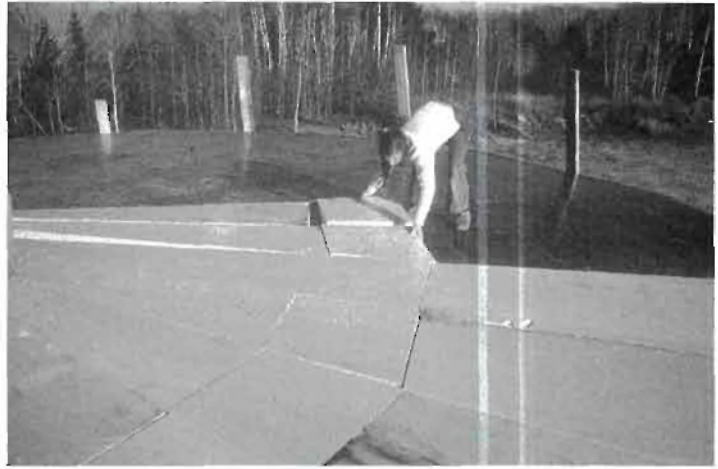
Fig. 7.12: Jaki installs the shiplapped insulation panels on the Earthwood roof.
