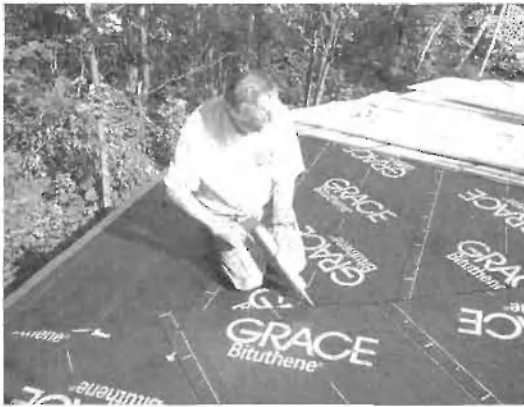
Fig. 8.1 (right): You can't see the clear "surface conditioner" which Grace provides with the Bituthene® 4000 membrane, but it's there and has dried to a tacky feel. Large trapezoidal sheets were installed first at the perimeter, lapping 2.5" onto the aluminum drip edge. Bruce Kilgore (left) and Darin Roy set a small trapezoid of Bituthene® 4000 close to the center of the building. Darin smoothens it down while Bruce pulls the backing paper off. We lap 3" onto the previous sheet and 3" onto the exposed planking. Therefore, there is always a 6" lap on the cut ends of the sheet.
