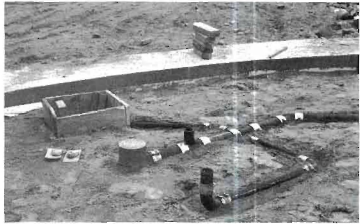
Fig. 4.9: Underfloor plumbing at Earthwood. The top of the cylindrical “red cap,” mentioned in the text, is set at finished floor level, which is the same as the top of the footings.
