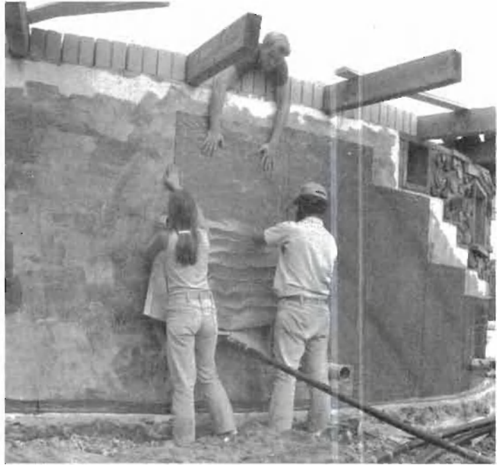
Fig. 7.2: Bituthene® waterproofing membrane is applied vertically to walls.
