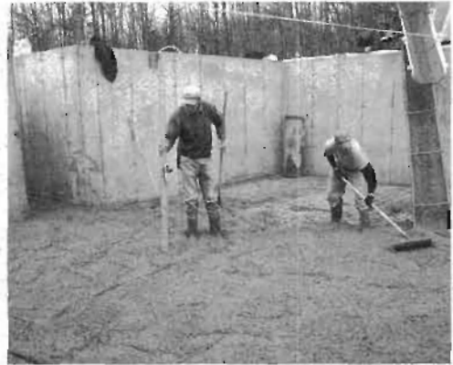
Fig. 4.14: The beam of a rotating laser level, 25 feet away, hits a grade stick. A benchmark on the grade stick shows if the concrete pad is high or low. Adding concrete or taking it away, brings the pad to finished floor level.
