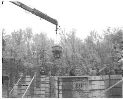
Fig. 5.1: Strong forms retain the concrete, which is delivered by chute, directly from the truck, or by hopper, controlled by the operator of the articulated boom.
