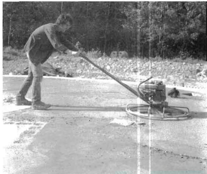
Fig. 4.17: Jonathan Cross power-trowels the slab at Earthwood.
