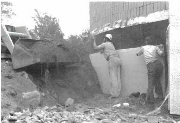
Fig. 7.10: “Bituthene® Protection Board Adhesive” for applying lightweight protection boards, such as extruded polystyrene, to the membrane. Grace warns, however, that the adhesive is extremely flammable and advises installers to read their Material Safety Data Sheet (MSDS), available at < www.graceconstruction.com >, before using it. Keeping an eye out for large stones, Jaki and Dennis hold the extruded polystyrene against the wall during backfilling.
