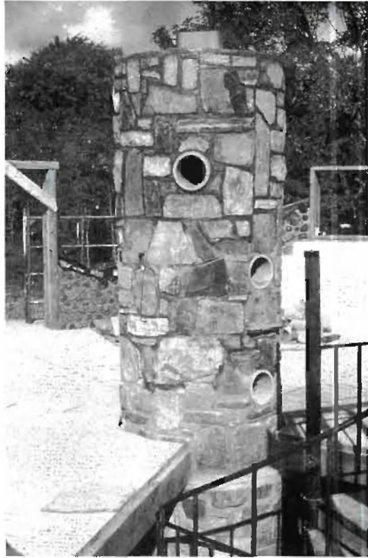
Fig. 10.3: The masonry stove at Earthwood.
