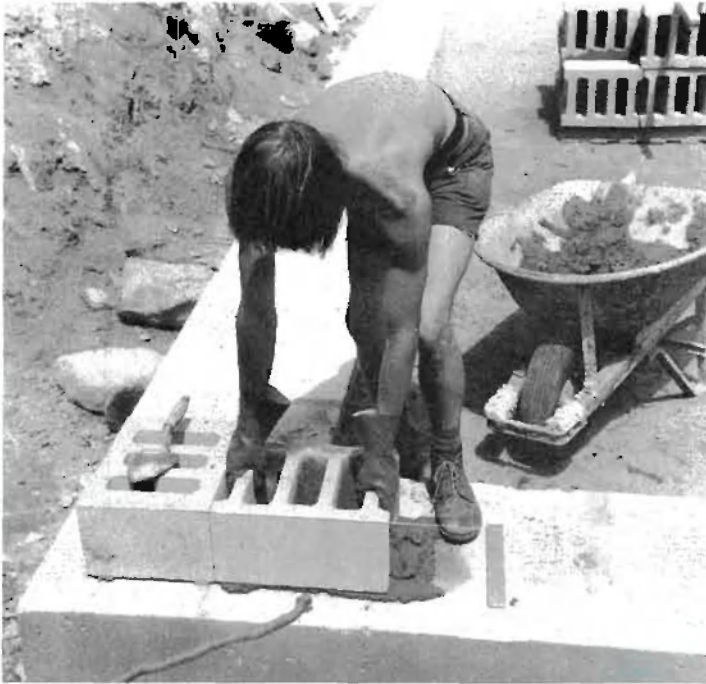
Fig. 5.3: The author lays the first blocks, in mortar, at Log End Cave, keeping blocks tight against each other.
