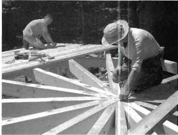
Fig. 6.18: Planking the roof at the Stoneview guesthouse was a lot like doing the Earthwood roof. Here, we snap a line on the planks, but directly over the middle of the 4 × 8" rafters. Next we cut off all the "waste" at once with a circular saw.
