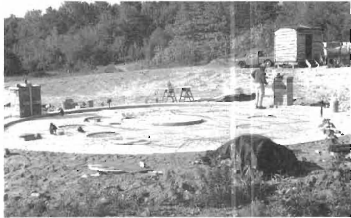
Fig. 4.5: Extruded polystyrene insulation and wire mesh are installed. The two buttresses are formed. We’re ready to pour!
