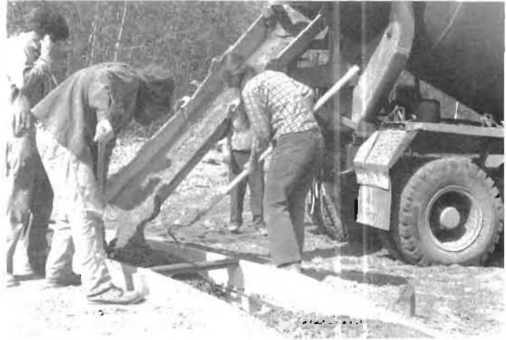
Fig. 3.22: Pouring the footings at Earthwood.
