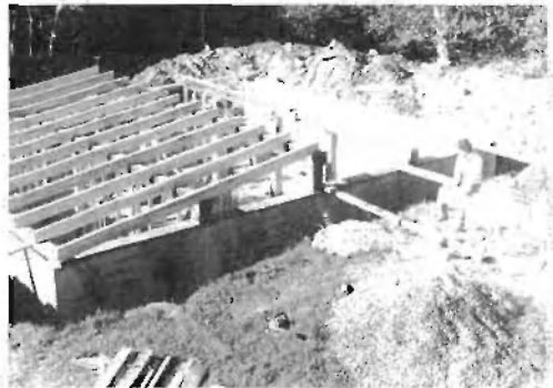
Fig. 6.9: Log End Cave, with half of the rafters in place.
