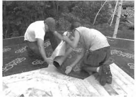
Fig. 8.1 (right): You can't see the clear "surface conditioner" which Grace provides with the Bituthene® 4000 membrane, but it's there and has dried to a tacky feel. Large trapezoidal sheets were installed first at the perimeter, lapping 2.5" onto the aluminum drip edge. Bruce Kilgore (left) and Darin Roy set a small trapezoid of Bituthene® 4000 close to the center of the building. Darin smoothens it down while Bruce pulls the backing paper off. We lap 3" onto the previous sheet and 3" onto the exposed planking. Therefore, there is always a 6" lap on the cut ends of the sheet.
