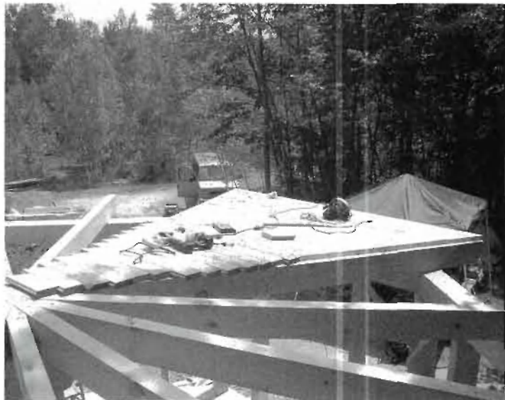
Fig. 6.19: The "waste" from the first cut is used further up the facet, so it isn't waste at all. Next, we would snap chalklines again and trim the two saw-toothed edges.
